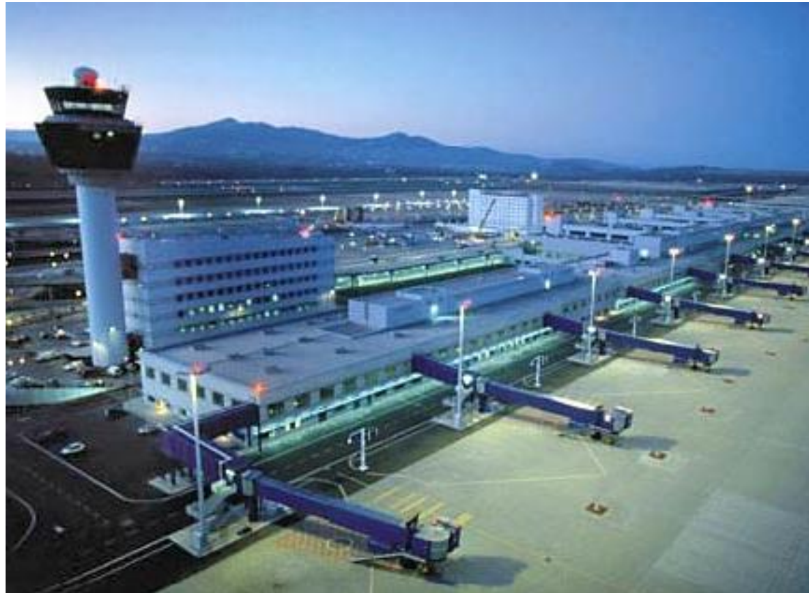
International Airport Athens: 4 x 450kVA
