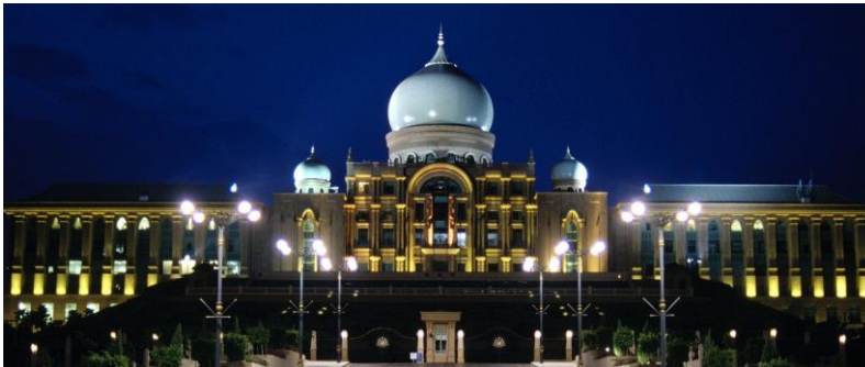
Prime Minister Office Putrajaya 1 x 1500 kVA (dual output)
