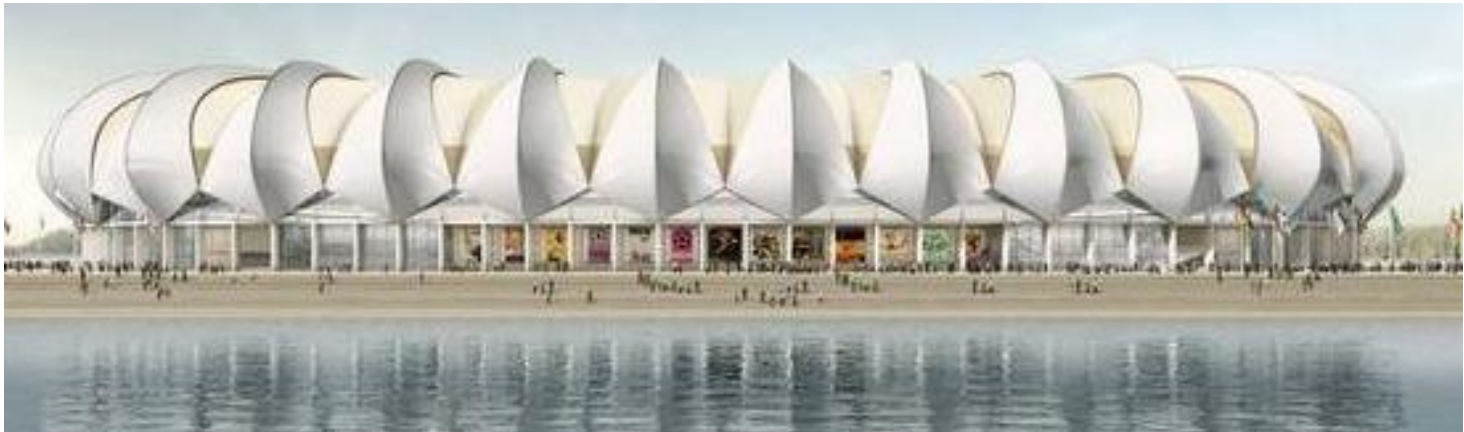
Nelson Mandela Bay Stadium - Port Elizabeth 4 x 550 kVA (dual output)
