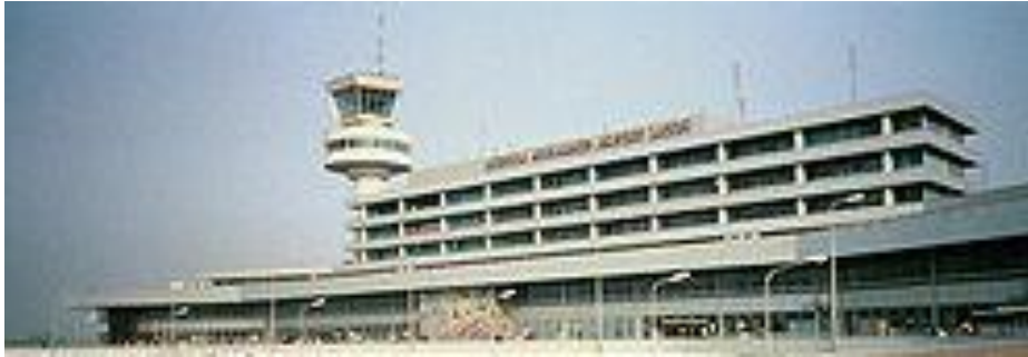
International Airport Lagos 2 x 250 kVA
