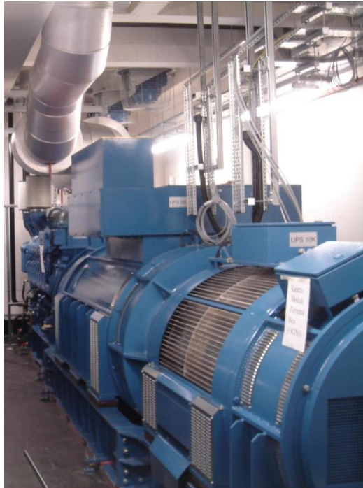
Data Centre – Global Switch London (22MVA in parallel Operation) 11 x 2000 kVA (11kV)
