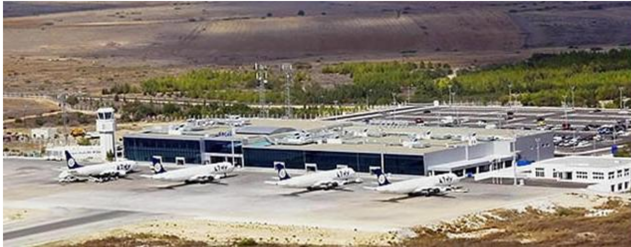
International Airport Lefkosa 1 x 325 kVA
