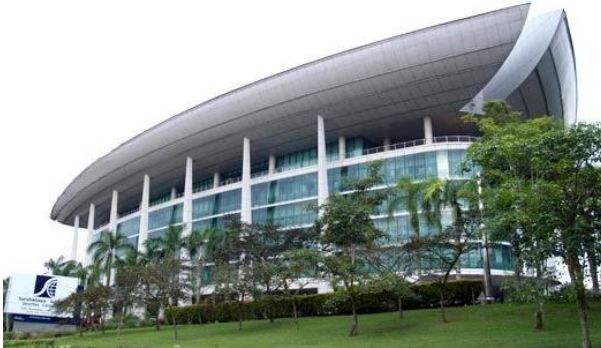
Securities Commission Building, Kuala Lumpur 2 x 150 kVA USV
